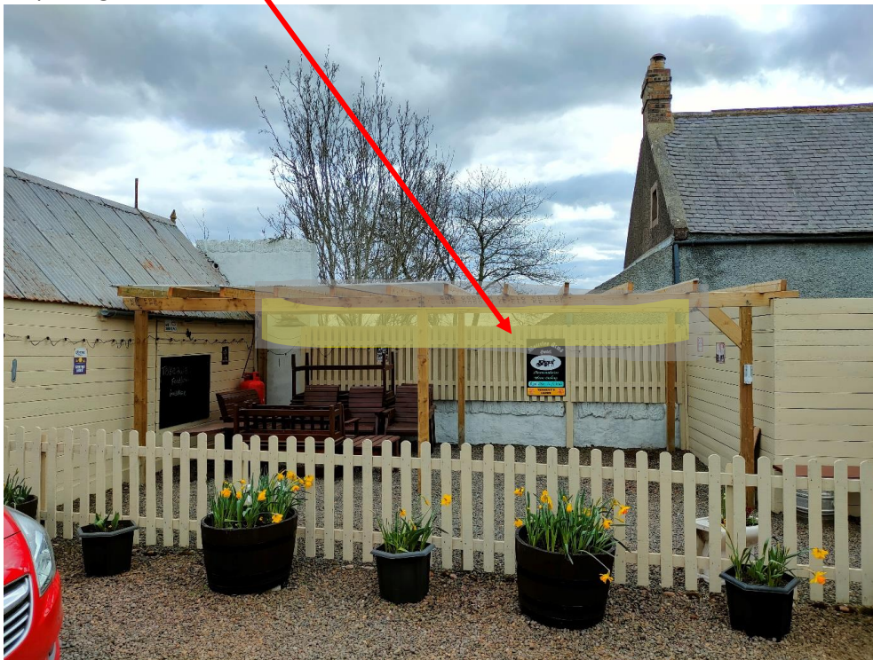
Existing Seating Area With Partially Completed Covered Pergola
